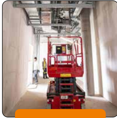
Fastening ventilation ducts
